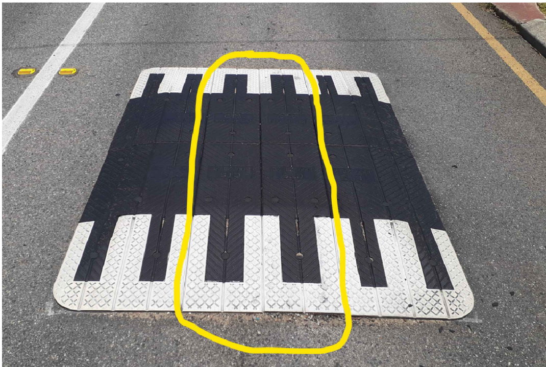
DETAIL B - REMOVED SPEED CUSHION MIDDLE SECTIONS
